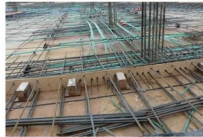
Steel cables laid along with reinforcement
