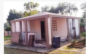
BRICK PYRAMIDAL ROOF
