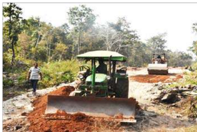
ROAD CONSTRUCTION ON D DAY
