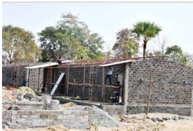
CONSTRUCTION OF BARRACK
