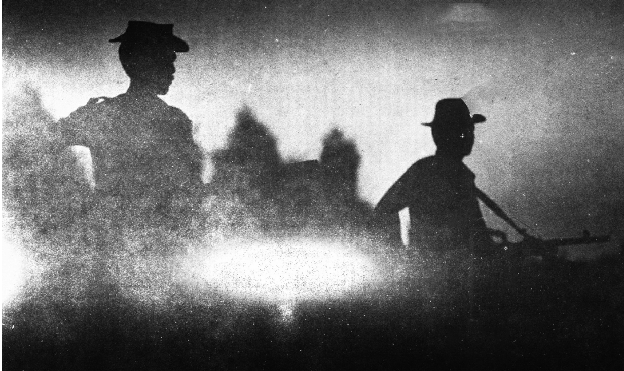
CRPF Personnel Clearing Operation Night Dominance
