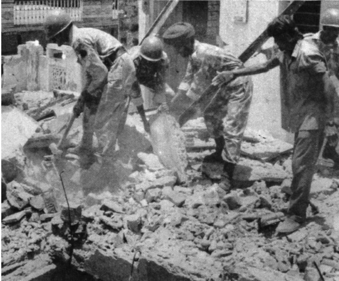
Rescue and relief work undertaken at the earthquake affected Jabalpur
